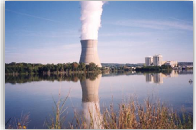
Industrial Water Supply
